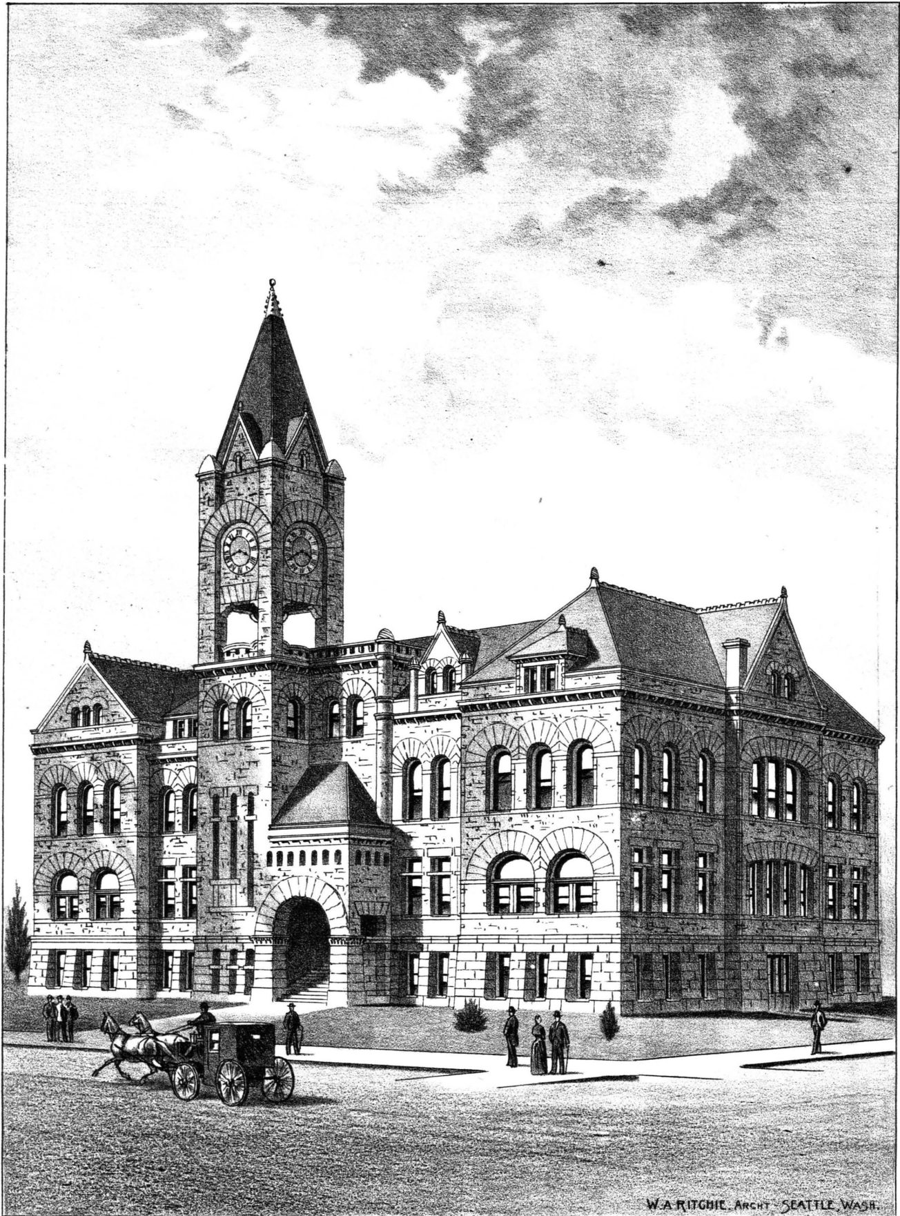
WASHINGTON—Court House at Whatcom. In course of construction—See Page 357.
